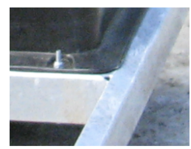
Float connection to steel
