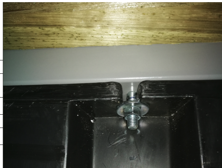
Steel frame-float connection
