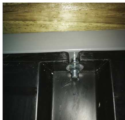
Connection of float to Steel frame
