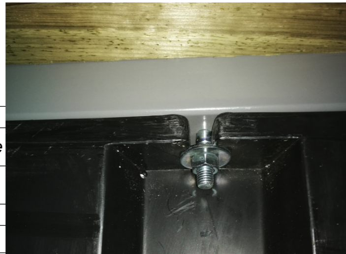
Steel frame-float connection
