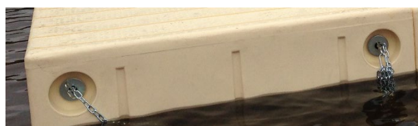
Picture 2: Fixing end of chain.
